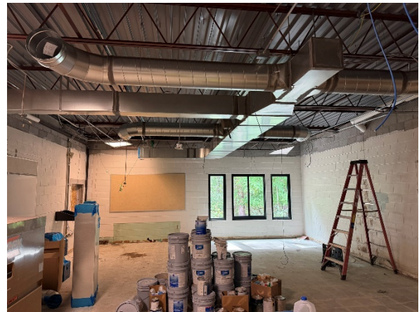
Phase 3 Classroom Mechanical Preparation
