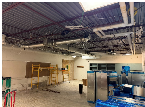
Phase 3 Ductwork Install
