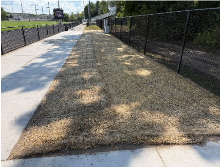
Football Field Sidewalk Relocation
