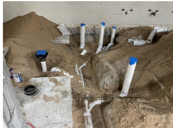
Phase 3 Bathroom UG Plumbing
