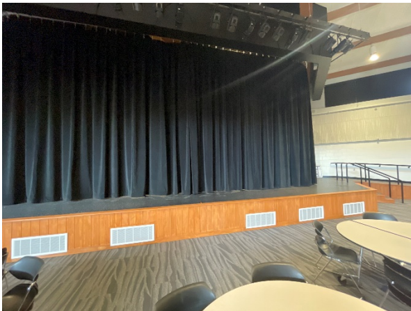
Cafetorium Stage Curtain Install
