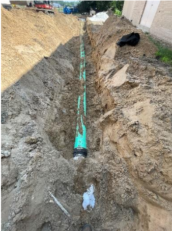
Storm Piping Replacements at High School
