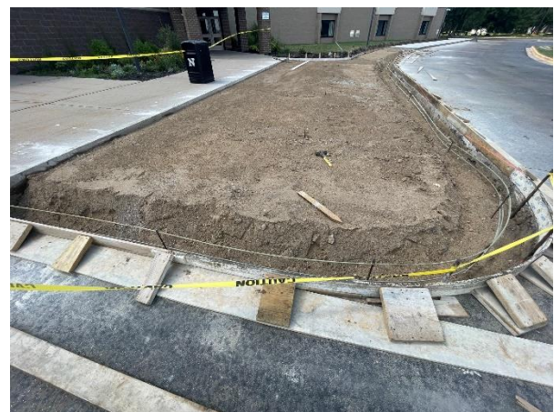
Completed Rebar Reinforcement Prior to New Sidewalk
