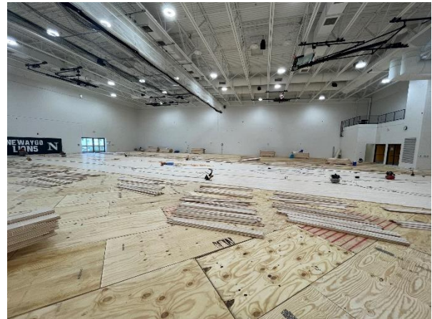
Wood Gym Floor Installation Progress
