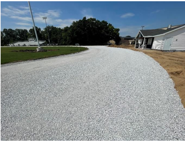
Track Final Sub Base Grading
