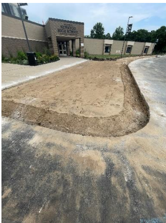
Demolition of Existing Failed Sidewalk
